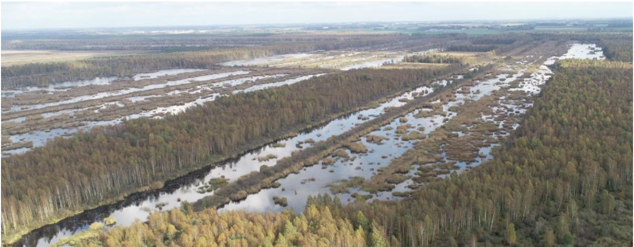
Ulila extraction area water treatment system (wetland / overflow area)
