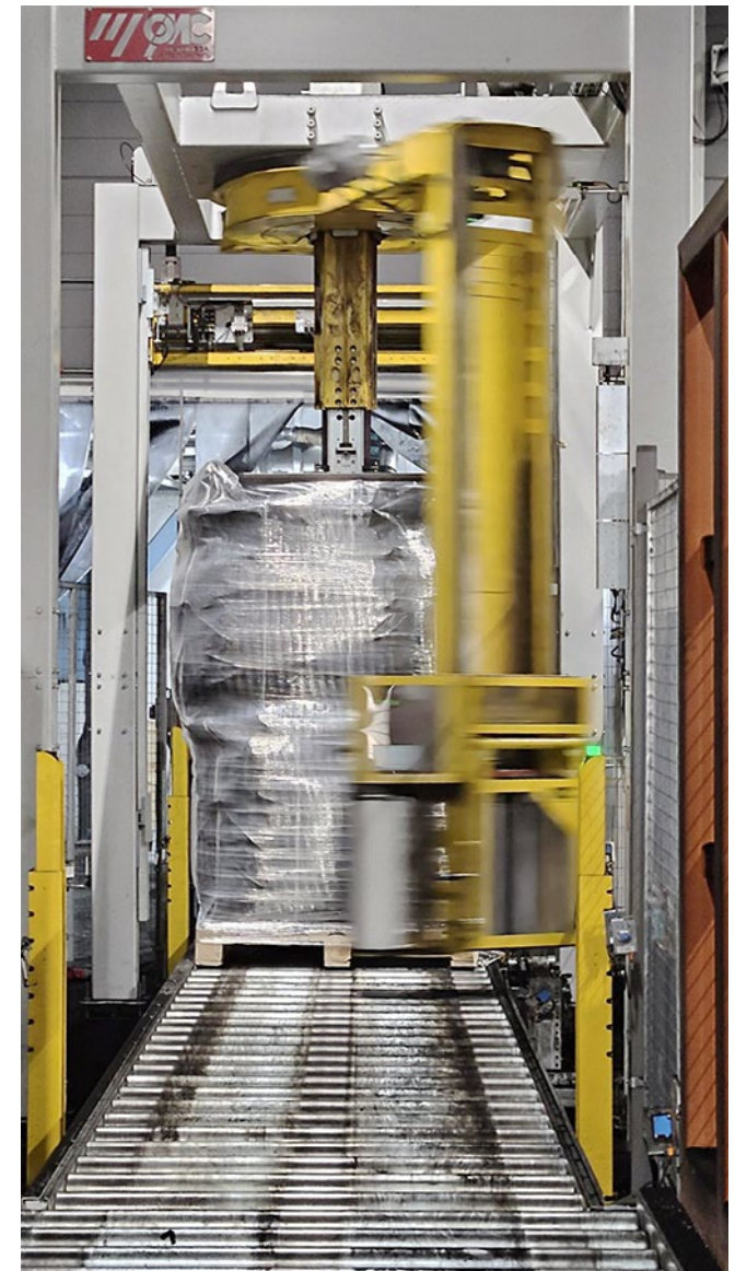
Automatic wrapping machine in operation at the Ilomantsi Activated Carbon plant.
